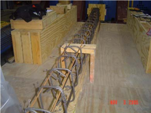
Fig. C-8: Rebar cage for prestressed beam.
