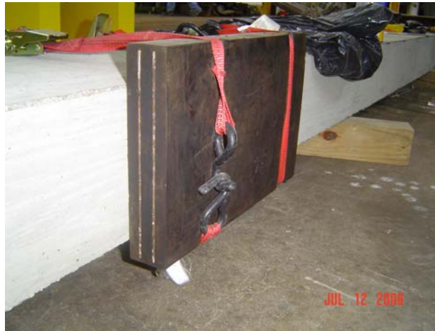
Fig. 5-1: Neoprene pad bonded to beam; straps are only used while epoxy sets.
