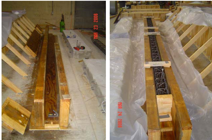
Fig. C-13: Formwork for reinforced concrete beam.
