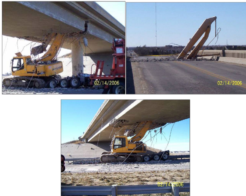
Fig. 2-4: Oversize load truck accident (source is unknown).
