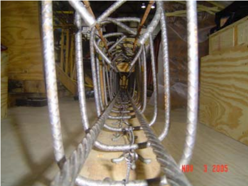
Fig. C-8: Rebar cage for prestressed beam.
