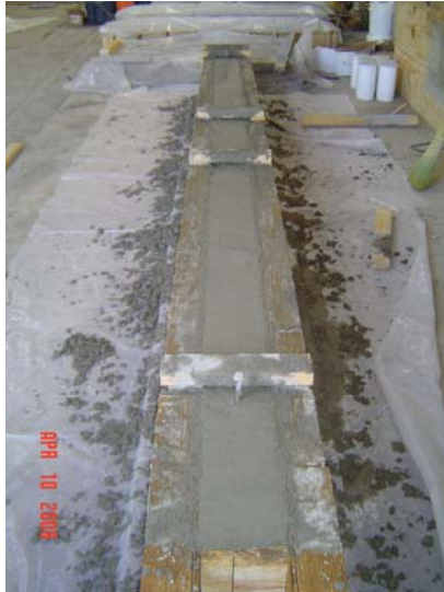
Fig. C-15: Placing of concrete for reinforced concrete beam.
