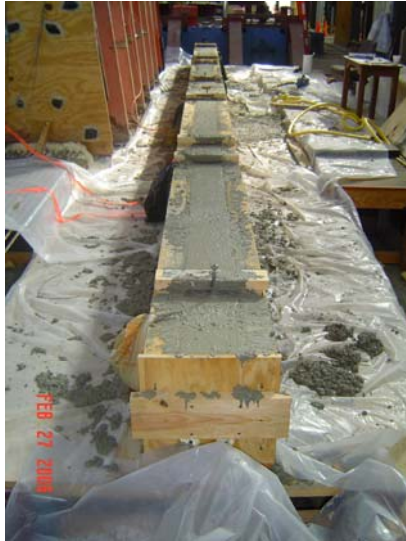
Fig. C-11: Pouring of concrete.
