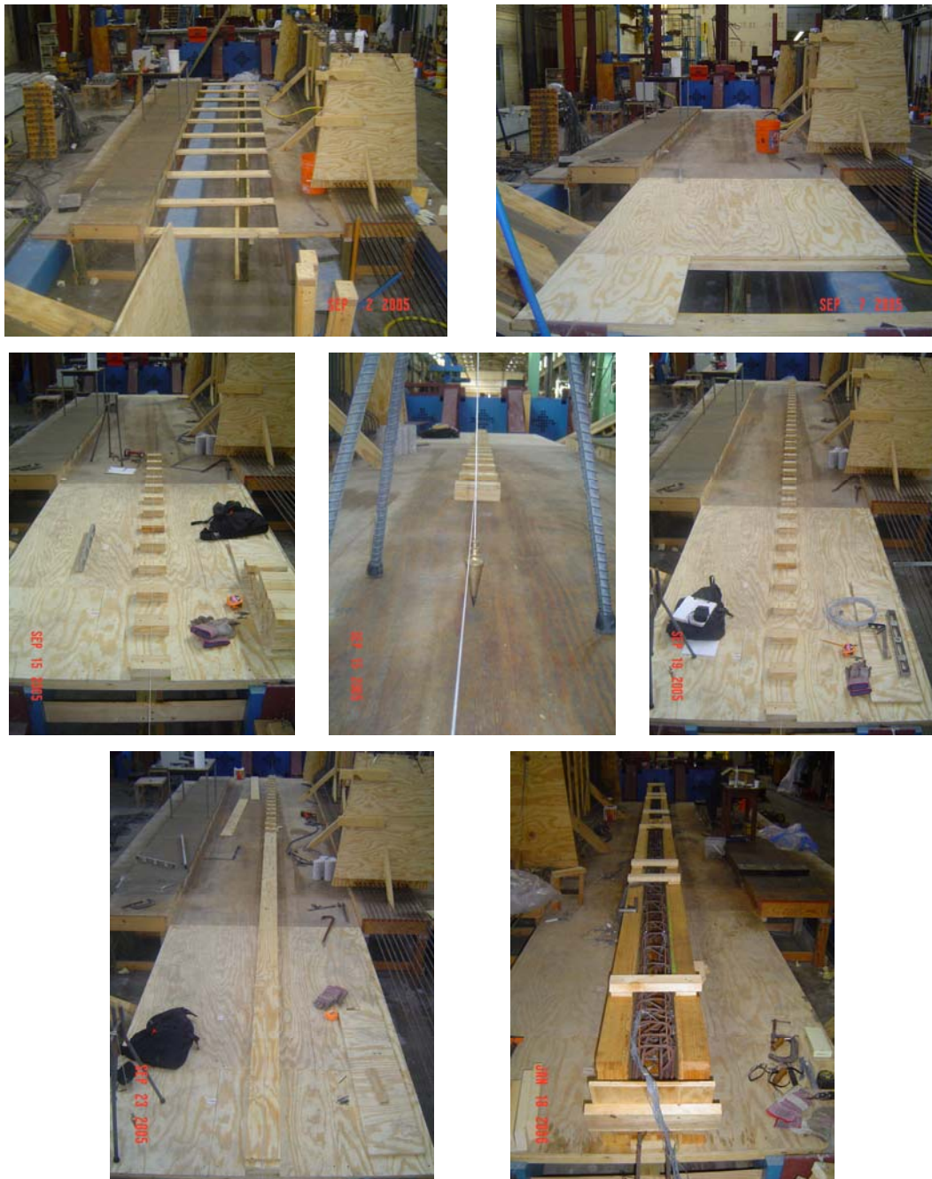
Fig. C-6: Formwork for prestressed beams.
