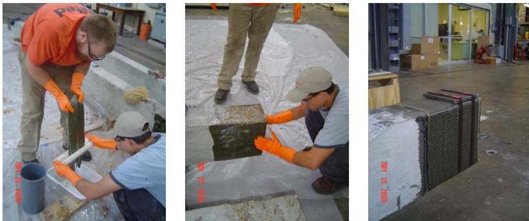
Fig. C-16: Placing FRP at ends of beam.
