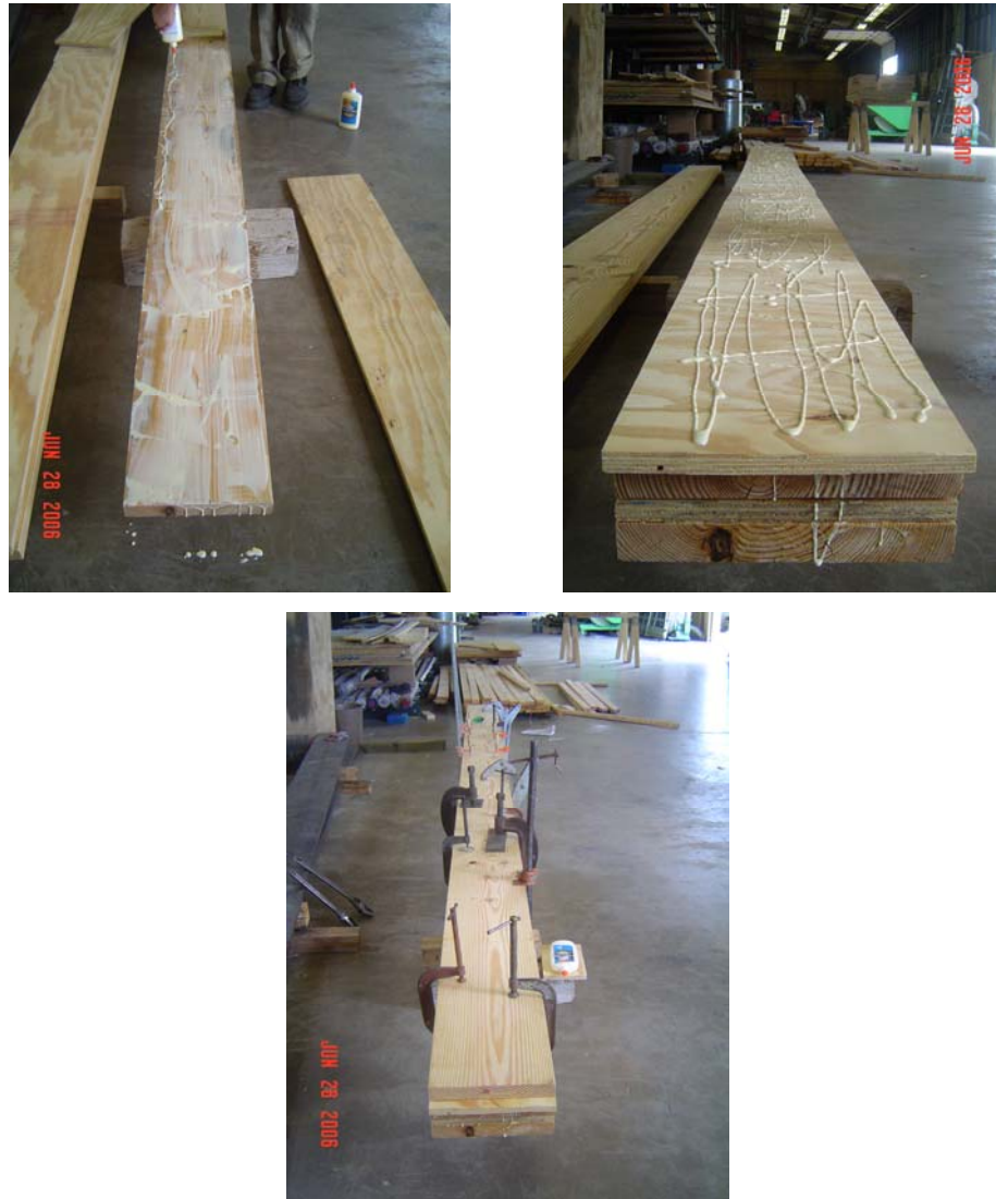
Fig. C-17: Fabrication of laminated lumber beam.
