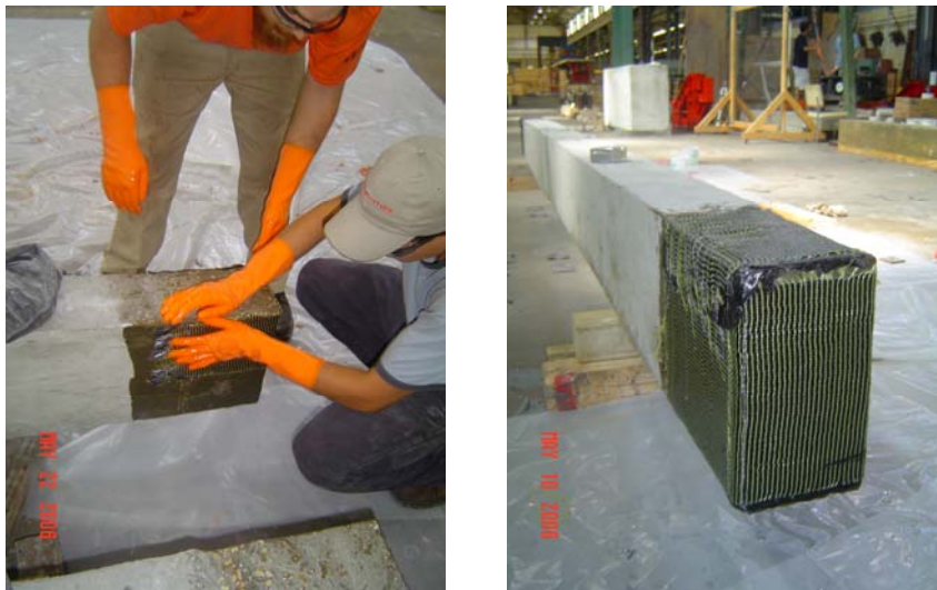
Fig. 5-6: Placing of FRP fibers on reinforced concrete beam.
