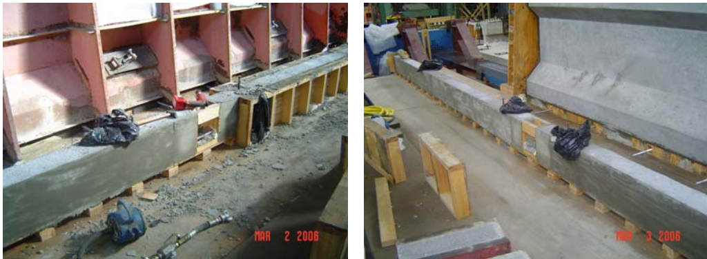
Fig. C-12: Stripping formwork.
